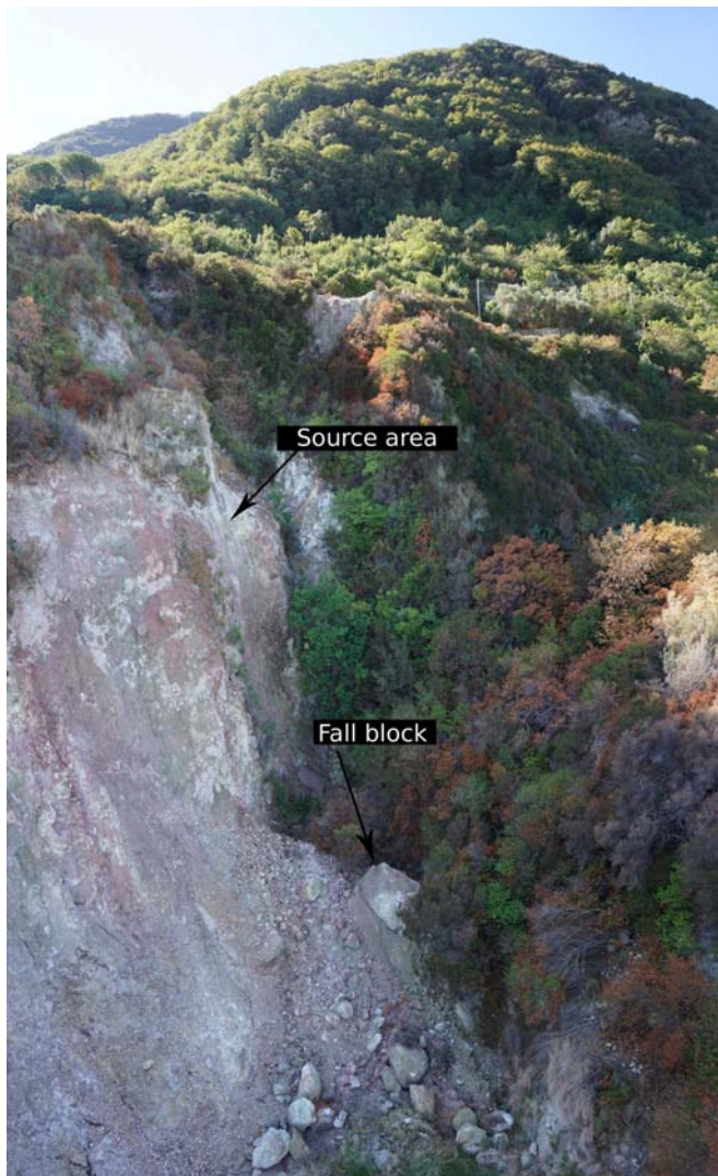
▲ Figure 6. Coseismic rockfall located in the impervious Pantane area by remotely piloted aircraft systems (Fig. 3 for location). The color version of this figure is available only in the electronic edition.
