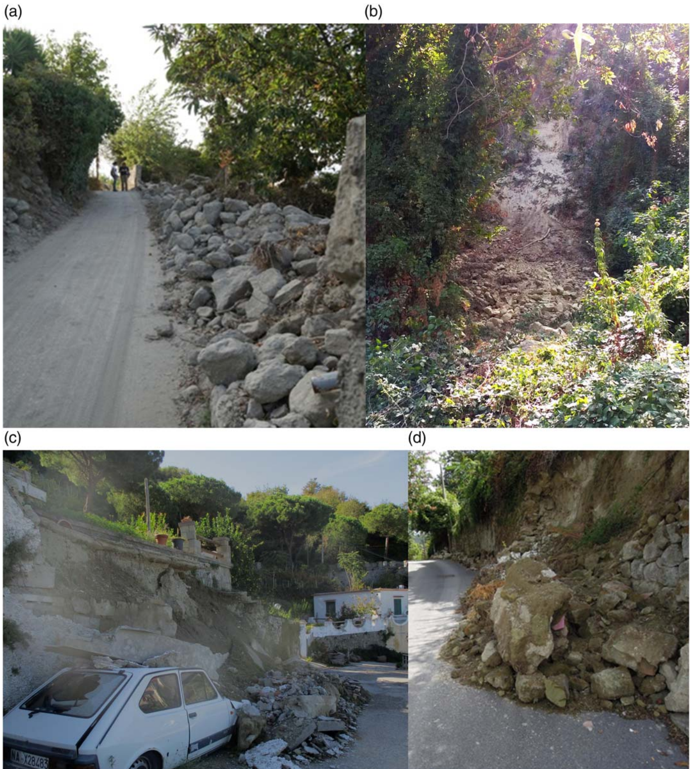
▲ Figure 8. The secondary coseismic effects observed: (a,c) collapse of drywall and man-made structure, (b,d) small rockfall and small debris flow in volcanoclastic deposits. The color version of this figure is available only in the electronic edition.
