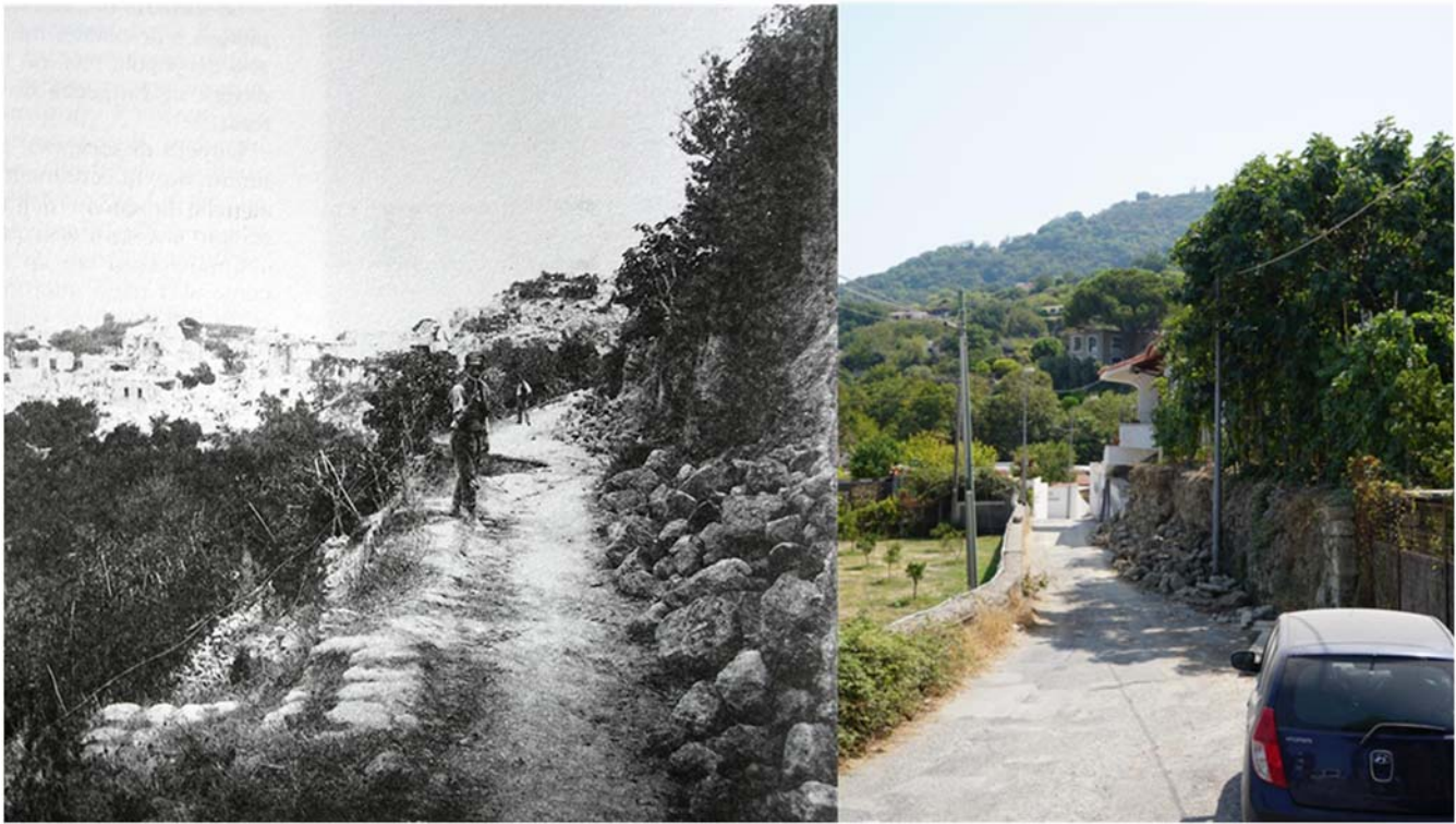
▲ Figure 9. Coseismic fractures and drywall collapses due to the 28 July 1883 historical earthquake along Campomanno road (near Santa Barbara locality) on the left (Ferretti, 1883), compared to the recent coseismic ground effects of the 21 August 2017 earthquake at the same location on the right. The color version of this figure is available only in the electronic edition.
