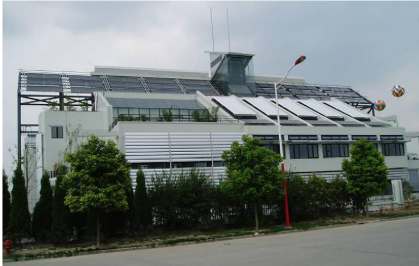
Figure 2: The installed solar cooling system in Shanghai.
