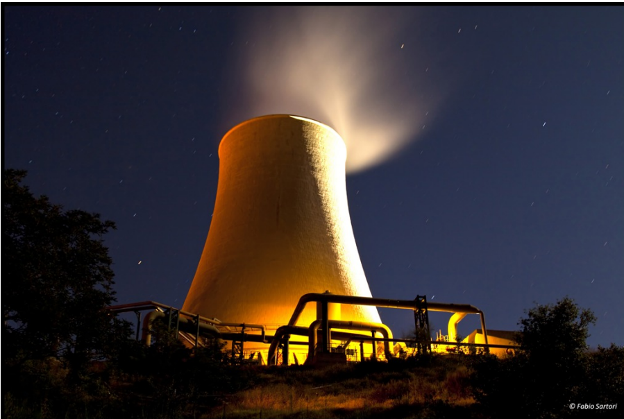
Figure 7. Nuova Monterotondo power plant natural draft cooling tower (photo by Fabio Sartori)
